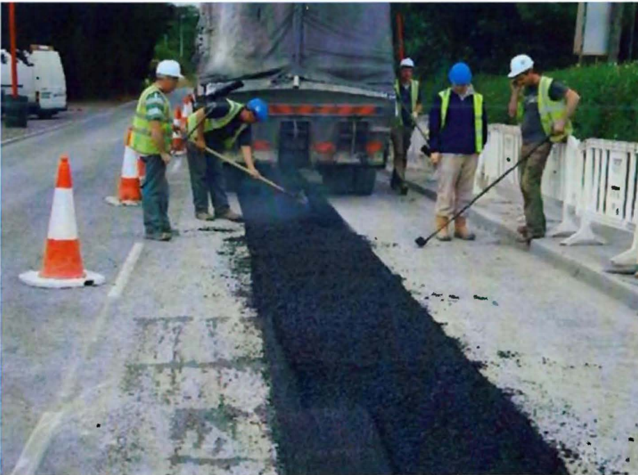
Figure 2.5: Reinstatement of Road Surface Over Trench
