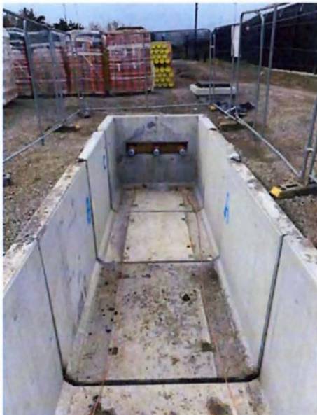
Figure 2.6: Completed Joint Bay prior to Cable Installation (pre-cast)
