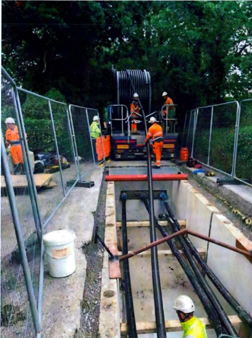
Figure 2.7: Typical Set-Up of HV Cable Pulling Procedure
